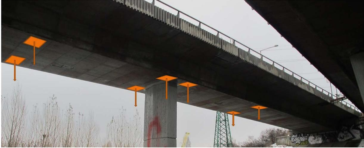
Figure 3: Vertical displacement determination of part of the Harbor Bridge in Bratislava
